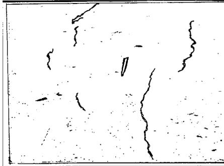
The most common reason why plastic shrinkage cracking occurs is because the evaporation rate of the water on the surface of the concrete is greater than the rate it is being replaced by bleedwater from underneath the surface. This situation will cause the concrete surface to shrink and crack even though the volume of the plastic concrete underneath the surface has remained the same.
